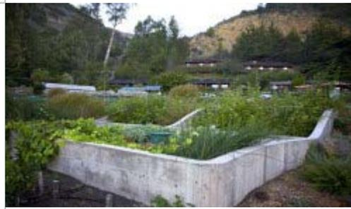
This "tidal-flow wetland" Living Machine treats wastewater from the laundry and lodging facilities at the Esalen Institute in Big Sur, California, for use in irrigation and aquifer recharge.
